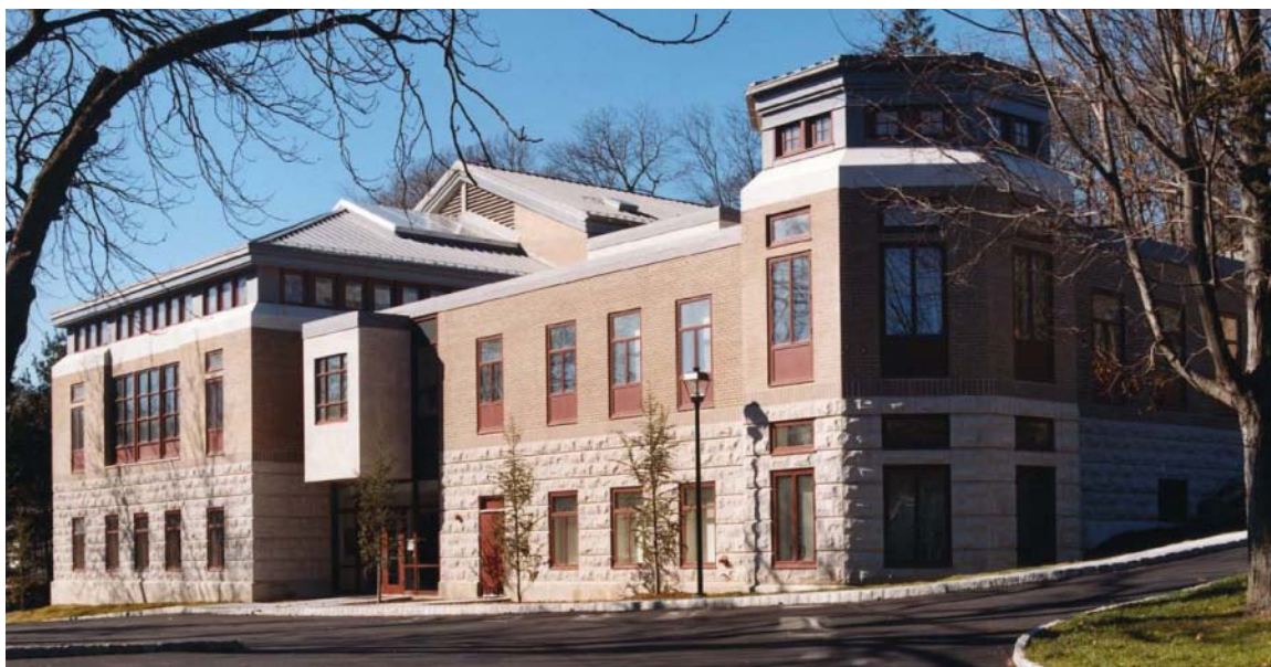
The John G. Rangos Family Foundation Building, which houses the seminary library, administrative offices, and the Metropolitan Philip Auditorium, was built through the generosity of benefactor John G. Rangos, Sr. and completed in 2001.
